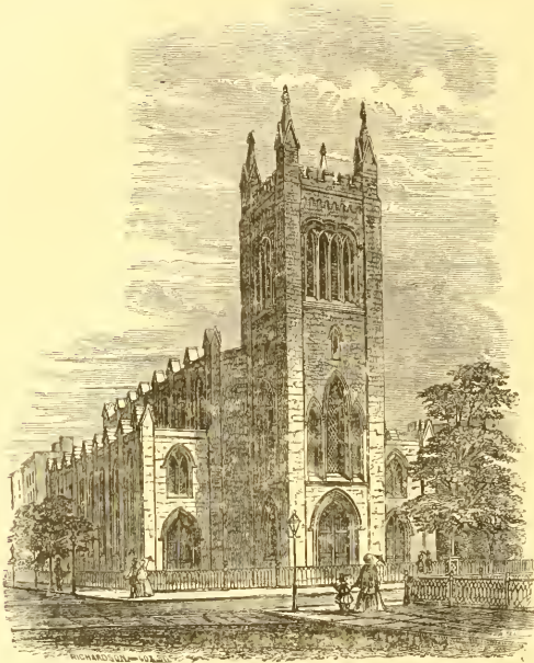
Church of the Ascension, corner of Fifth Avenue and Tenth Street.
